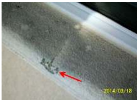
Repair bull nose sill damage.
