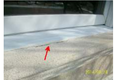
Gaps at flat window sills can allow for moisture to enter the wall assembly.
