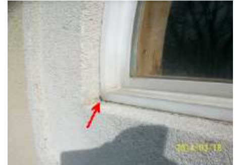
Gable window has never been sealed.
